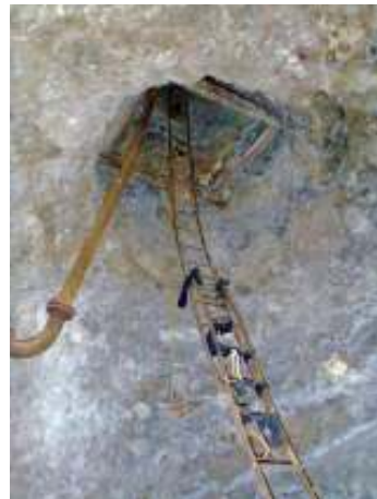
Figure 8: Long ladder leading into a shaft (about 50 ft overall). Note the use of rags to tie two sections of ladder together to reach the desired height.
